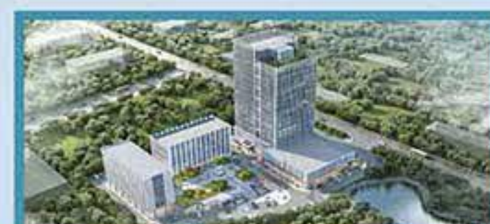
R&D Center in Wuhan
